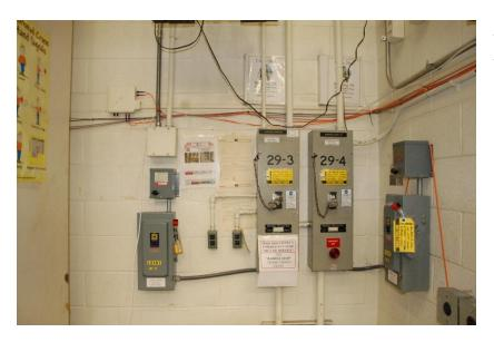
Crane power switches, main power disconnects, RECERT tags and log books are typically located together.
